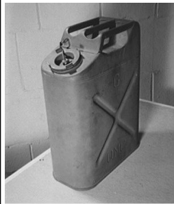
The original German "Blitz" can, built w/ handles for two to carry. Photo Library of Congress
